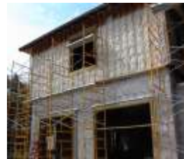
Exterior cavity-wall installation = air barrier continuity
