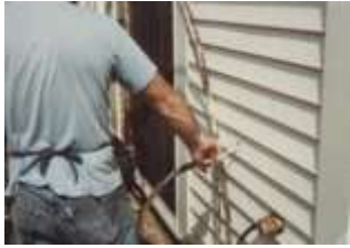
Using kit foam to seal small bays
