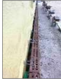
Exterior cavity-wall installation = air barrier continuity
