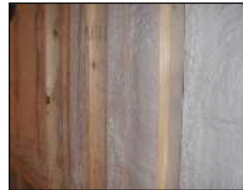
Closed-cell in a double 2x4 Wall - R-21 with no trimming
